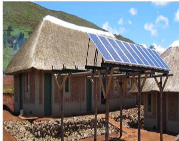
Fig. 4 Rural electrification project based on a standalone home energy system
